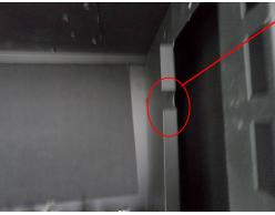
NOTE: It is recommended to use two people to remove the glass. There are two holes at each side behind the mirror glass. You can put your finger in and take out the glass. You can use one hand to lit up the up panel let the glass easy to be taken out.
