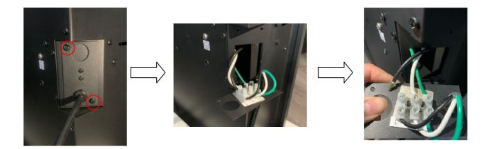
2. Cut off the copper head of the wiring and leave 1 cm (0.4 inch) uncovered wiring.
